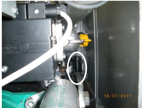
Figure 9.2 - Water Flow Switch
