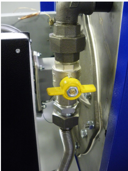
Figure 7.2.1 - Gas Isolating Valve (97 & 116 shown)
