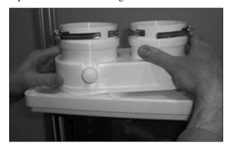
3) Rotate the New Adaptor (Clockwise) until it clicks into place (less than ¼ turn) and is square with the front of the Challenger.
