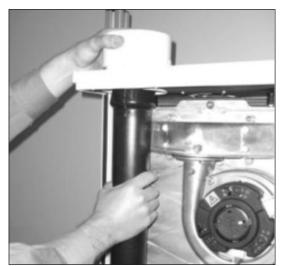
3. Remove the o-ring from the adaptor. Save this oring to be installed onto the New Adaptor.
