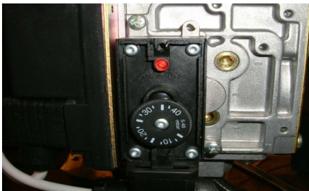
Fig 7.3.2 - Low Gas Inlet Pressure Switch
