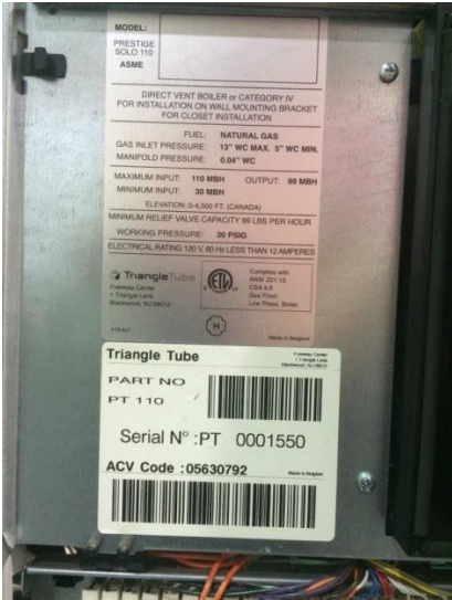
Prestige Trimax Boiler rating label with Serial Number
