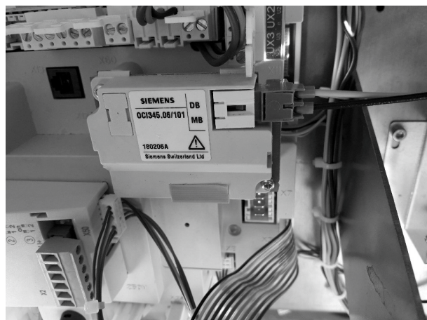
Figure 3: Screw Terminal Connector inserted into OCI345 unit
