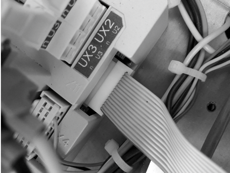
Figure 6: Terminate ribbon cable into LMS Controller
