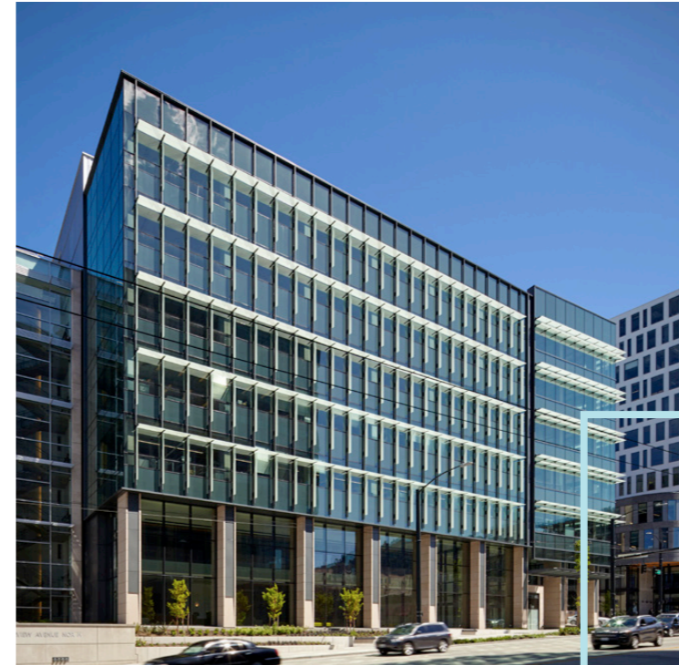
Vue Research Center, Seattle, WA
