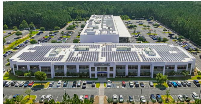
Solar installation at Gulfstream’s Savannah Research and Development Campus
