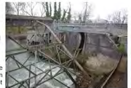
Photo 4 – Avon Mill Radial Gate
