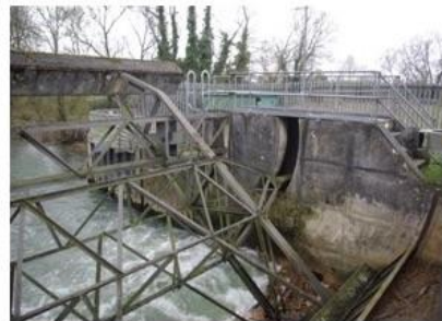
Photo 4 – Avon Mill Radial Gate
