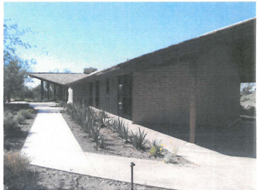
The strong north-south axis of the house, with the extended overhang on the south side and the flared-up roof on the east side captures views of Camelback Mountain
