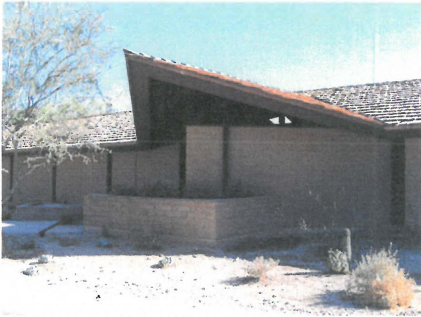
The swept-up roofline on the east creates the entrance
