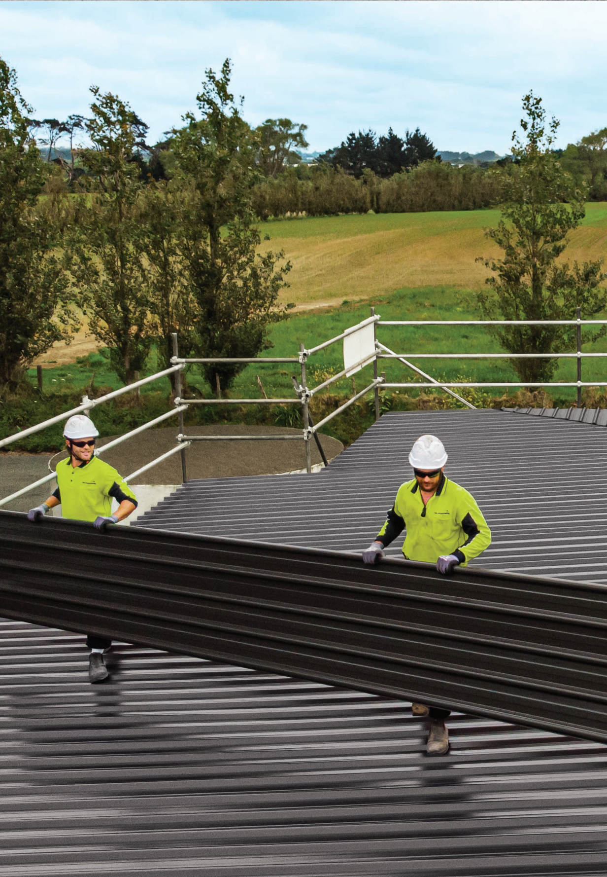
With no need to lay separate underlay, COLORSTEEL DRIDEX® can be installed in 90% of wind conditions
