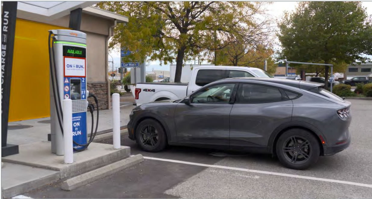
First ON the RUN EV charging location: Kelowna, BC (September 2021)
