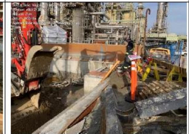
Safe means of access and egress
