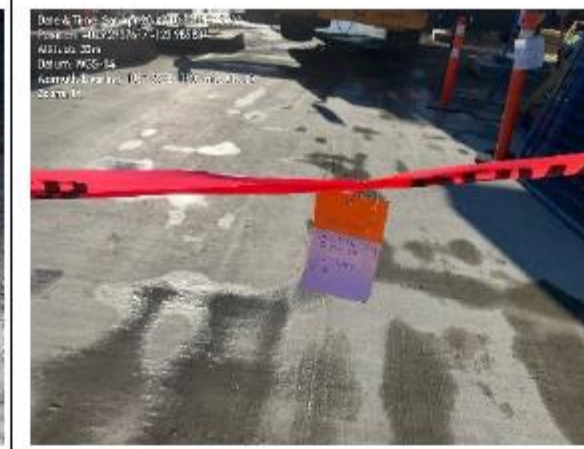
Warning tape to secure work area
