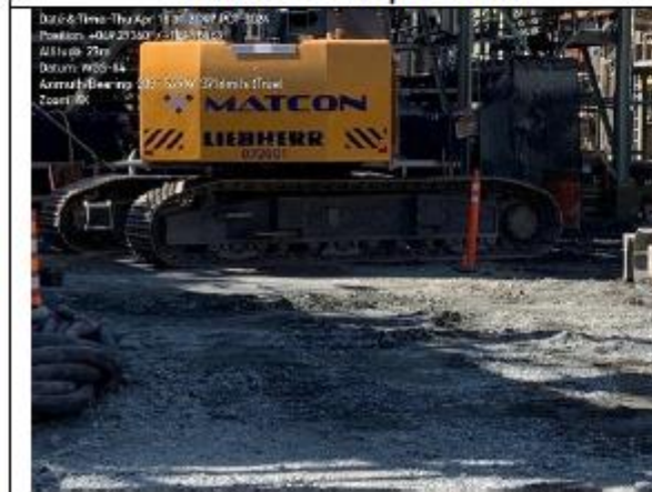
Leveled and repacked the walking area
