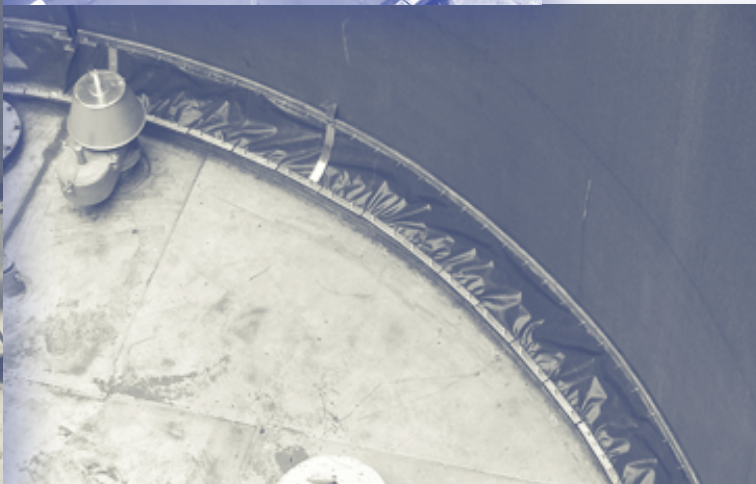
FLOATING ROOF TANKS ARE EQUIPPED WITH SECONDARY TANK SEALS
