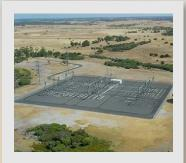
**Grid Connection Landwehr Power** Terminal / SWIS 33/330kV transformer 3.5km from BSS
