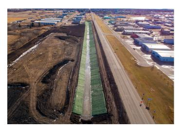
was conducted upstream, within, and downstream of the **PROPEX** Pyramat-lined drainage channel, which was initially installed in 2021. Two years after the installation, the tests revealed that the water downstream of the **PROPEX** Pyramat showed a considerable reduction in heavy metals and total suspended solids (TSS) levels compared to the water in the upstream, unreinforced section.
