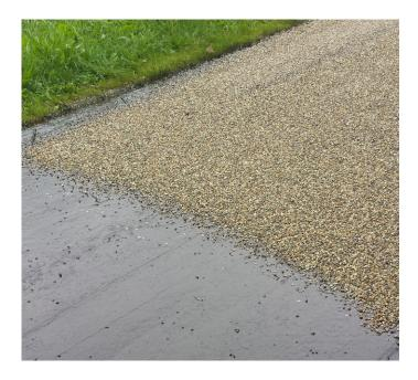
The aged bitumen created a cracked surface that allowed water to penetrate the road construction. This was an ideal scenario for applying **MIRAGRID** PGM 14 in combination with polymer modified bitumen. The installation of 3,000 m<sup>2</sup> (32,292 ft<sup>2</sup>) of **MIRAGRID** PGM 14 took only a few hours, allowing the entire project, including double surfacing treatment, to be completed in just one day.
