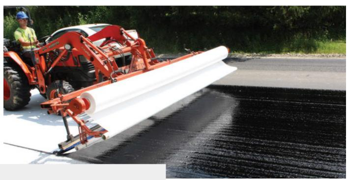
Petromat Enviro provides unmatched moisture protection for roads while absorbing stress to slow fatigue and reflective cracking in asphalt pavement. This patented interlayer solution outperforms the competition from start to finish.
