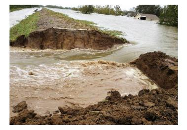
of risk reduction. One of the most critical measures of the HSDRRS was the protection of refurbished earthen levees against the erosion-causing hydraulic forces of storm surge overtopping. Without protection, overtopping can lead to significant landside erosion and potentially a breach of the levee. During Hurricane Katrina, most levee failure was due to water overtopping.
