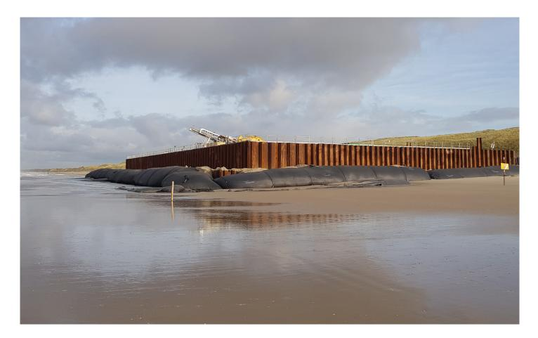
Industry:EnergySub-industry:WindLocation:The NetherlandsProduct:GEOTUBE® Marine
