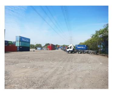
reduced base course thickness of 500 mm (19.69 in) provided a stable load supporting platform for container handling and storage. This geotextile offered reinforcement, base course confinement, separation, and permeability, effectively improving subgrade stabilization. The solution proved to be cost-effective compared to the initial construction without geotextile, which was both expensive and unsatisfactory.
