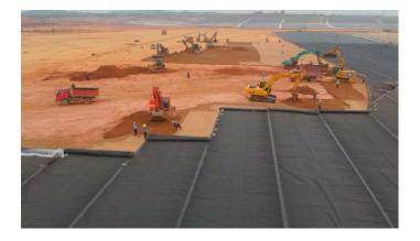
After the new stack pond was put into use, Shanghai Shengyi commenced work on the safe storage of phosphogypsum in the old pond and gradually completed its ecological restoration. This restoration included the use of ultra longdistance horizontal directional drainage technology, deepburied vertical gas-driven technology, an ACL artificial barrier liner, ecological-solidification liner, and other materials.
