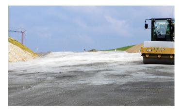
**MIRAFI** Geolon PET 800 geotextile reinforcement, with an initial tensile strength of 800 kN/m (456 lb/ft), fulfilled the long-term design requirements and was subsequently used for the basal reinforcement.
