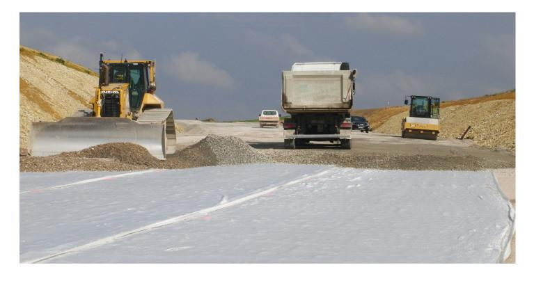
Industry: Application: Location: Product: Transportation Reinforcement over cavities Germany **MIRAFI**<sup>®</sup> Geolon
