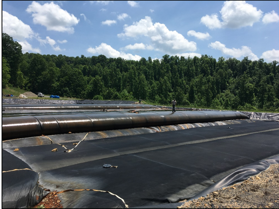
Figure 5 Geotextile tube dewatering cell
