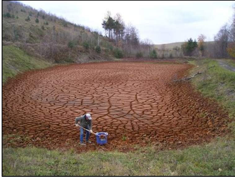
Figure 3 Typical AMD high moisture content “red mud” filled lagoon
