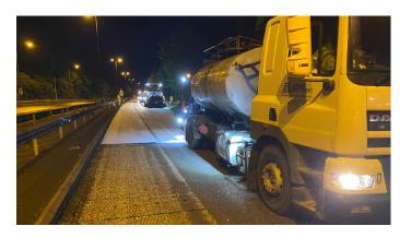
the supply and installation of asphalt Geosynthetics. AGS chooses to use **MIRAGRID** PGM-G 100/100. M products based on their long experience. These products are specially designed for asphalt pavement applications, including new road construction and the rehabilitation of existing roads, complying with EN15381.
