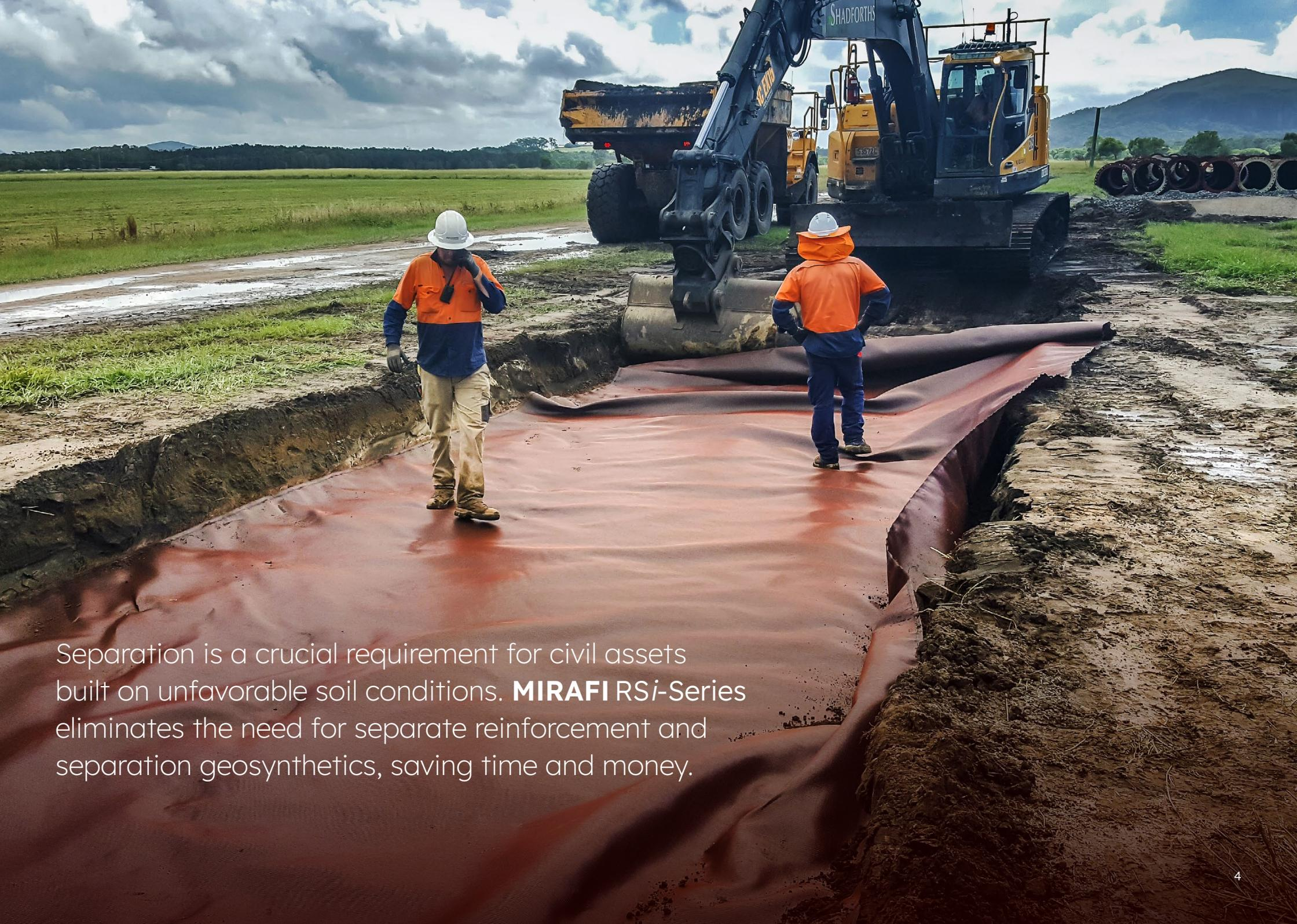
Separation is a crucial requirement for civil assets built on unfavorable soil conditions. **MIRAFI RSi-Series** eliminates the need for separate reinforcement and separation geosynthetics, saving time and money.
