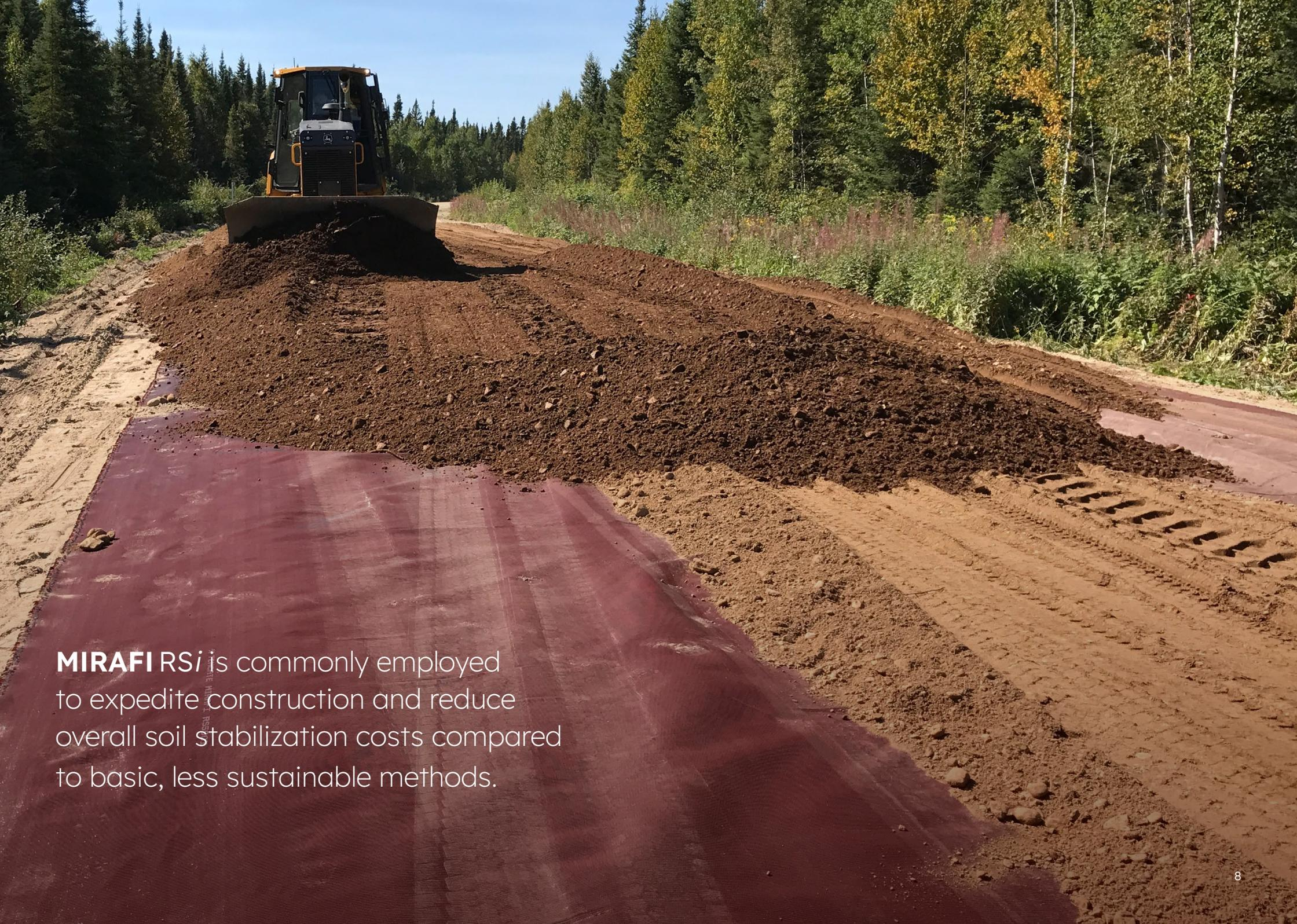
**MIRAFI RSi** is commonly employed to expedite construction and reduce overall soil stabilization costs compared to basic, less sustainable methods.
