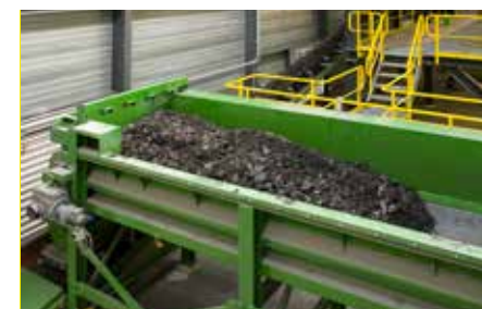
Bitumen recycling Groningen (NL)
