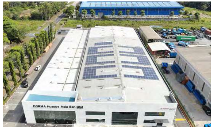
Operation centre of dormakaba Group in Senai, Malaysia, with solar panels.
