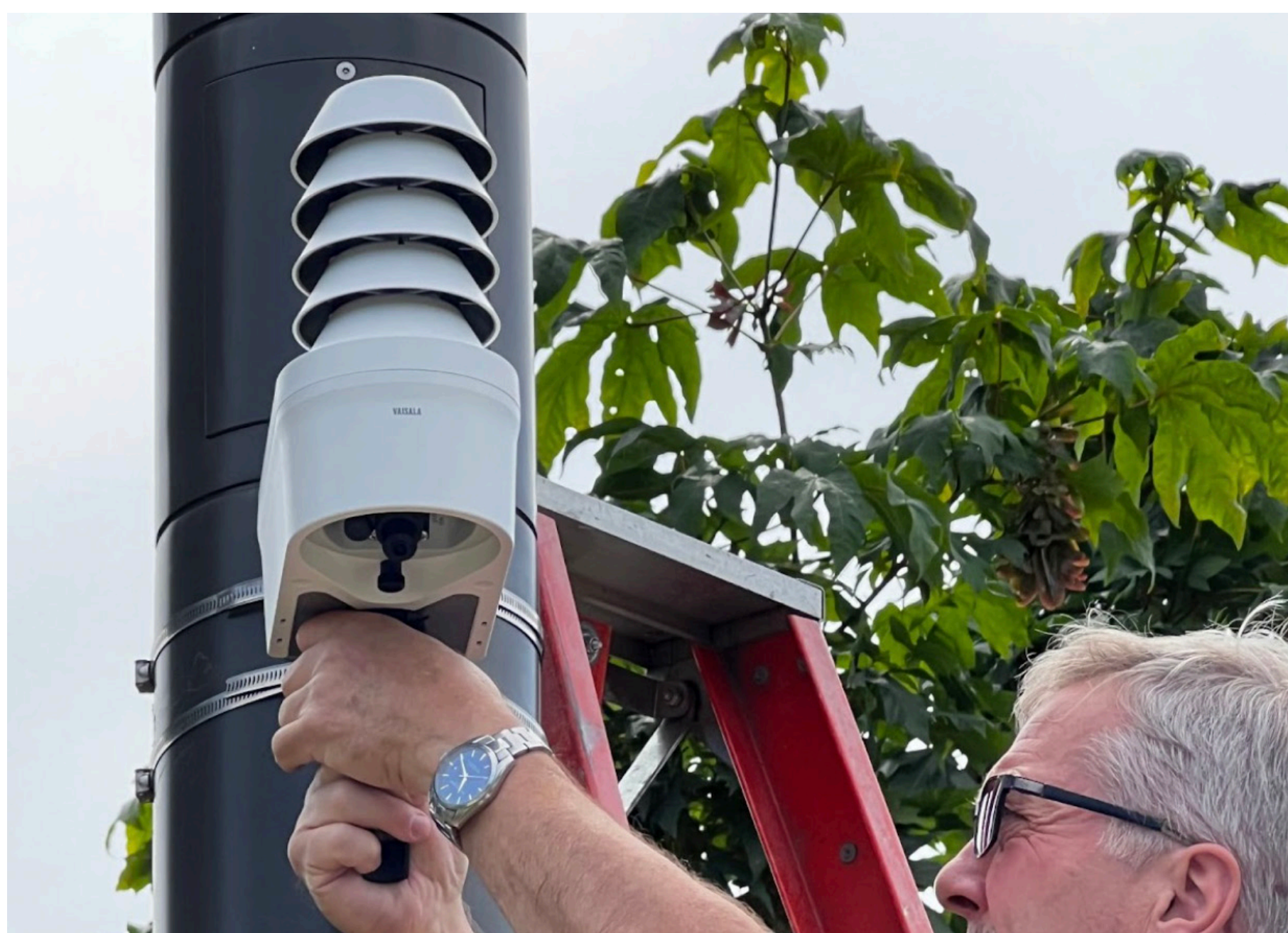
Installing Tempcast sensor
