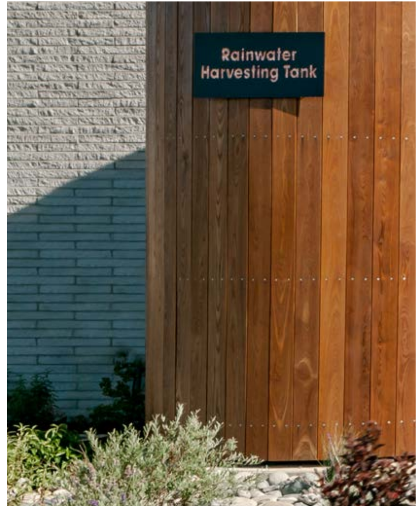
The Columbia Credit Union, completed in 2020, features a rainwater harvesting tank.
