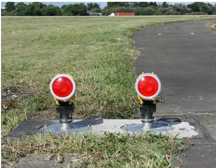
Elevated Stop Bar.
