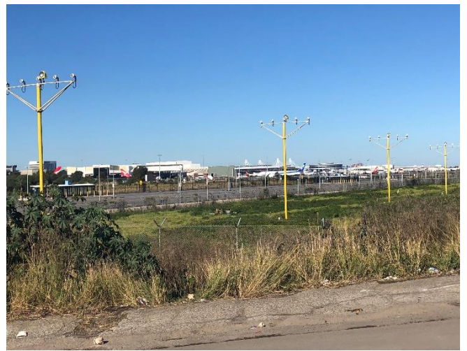
Figure 19.8 High intensity approach lighting
