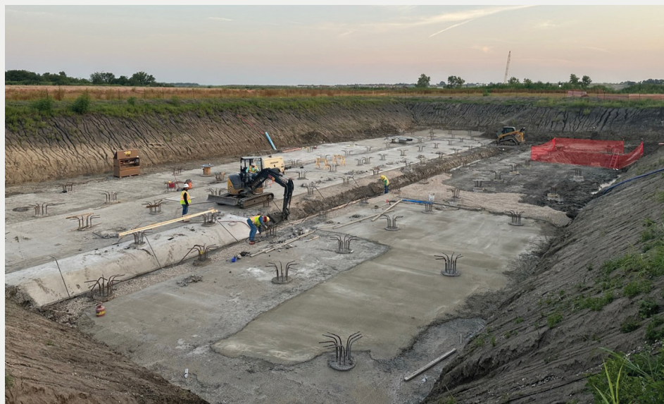
Piers are being drilled to solidify the foundation of the pump station.
