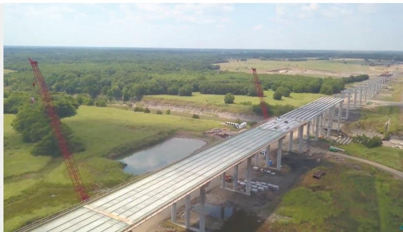
Construction is installing the last of the 343 large, 125-foot-long beams this summer. Merrill Creek Bridge, a second bridge that will offer access over a finger of the lake, is also underway with columns being placed and beam installation continuing in the coming months.
