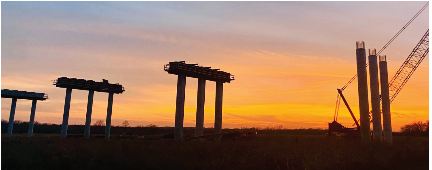
Columns are going up to support the future SH 34 Bridge over Lake Ralph Hall.
