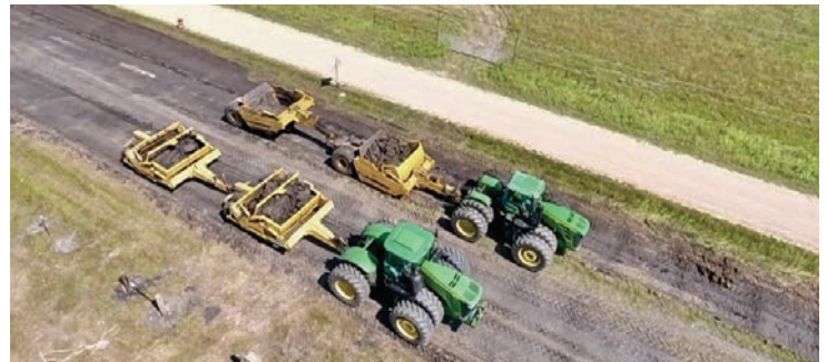
Site grading for the relocated FM 1550.
