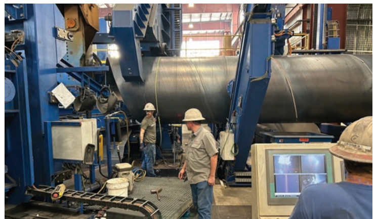
Manufacturing of pipeline for the lake project.
