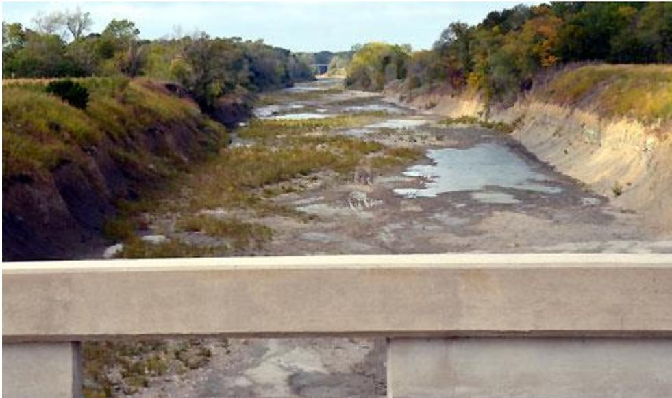
Erosion has transformed a relatively miniscule 16-foot wide, 10-foot deep channel that was excavated in 1928-29 into a 300-foot wide channel that continues to erode. *photo by Allen Rich*
