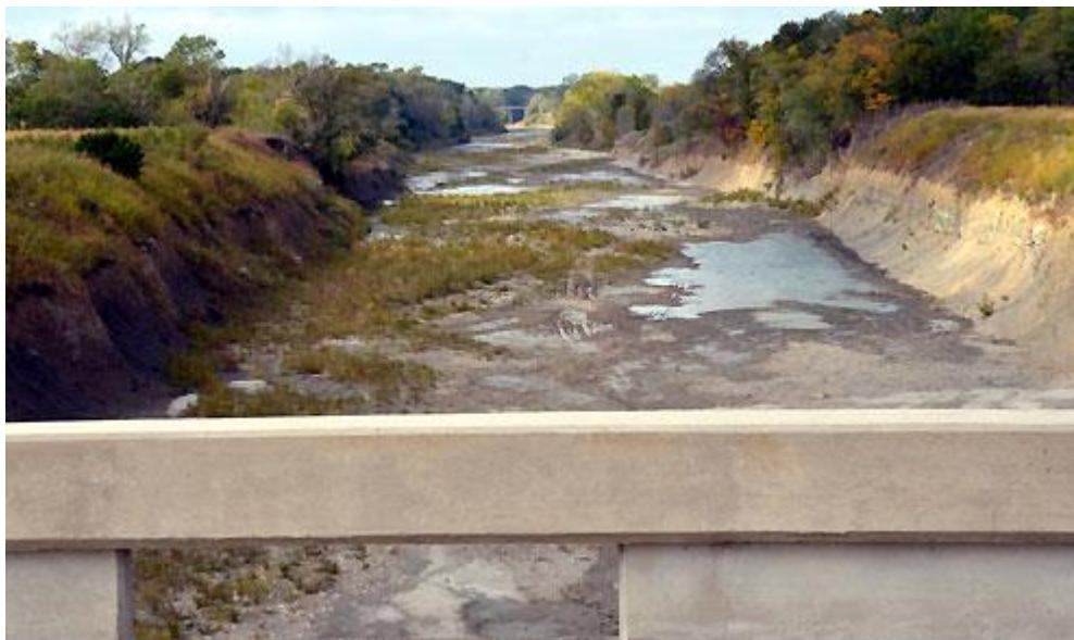
Erosion has transformed a relatively minuscule 16-feet wide, 10-feet deep channel that was excavated in 1928-29 into a 300-foot wide channel that continues to erode. *photo by Allen Rich*
