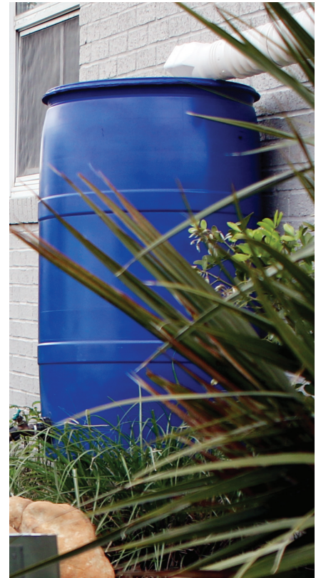
A food-grade rain barrel at Water University's WaterSense Labeled home sits slightly taller than a window sill.
