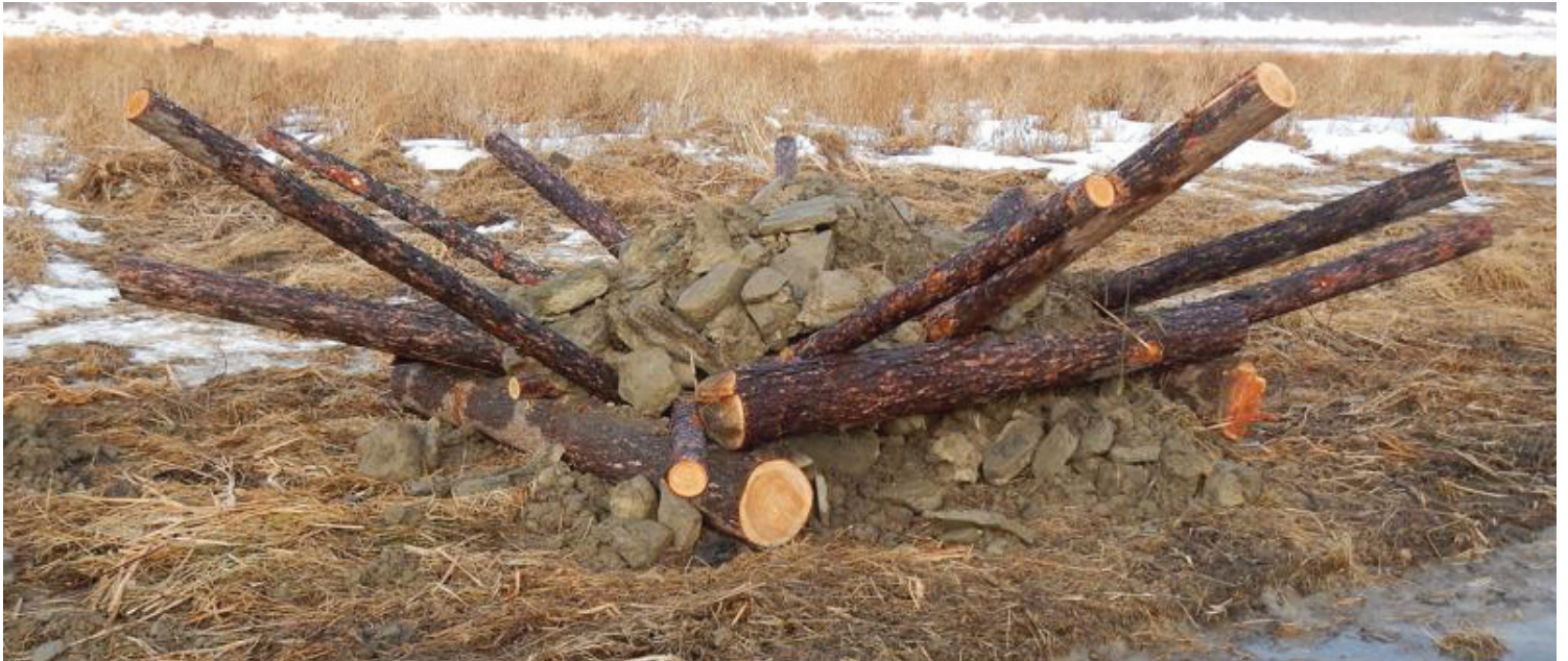
Example of fish habitat that will be built from cut timber in the lake footprint.
