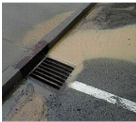
Figure 4. Stormwater runoff entering a storm sewer, which may discharge directly to a stream.
