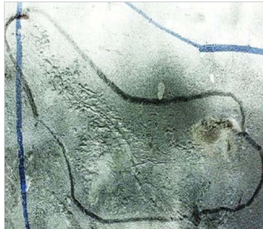
Axial crack colony surrounding the dent
