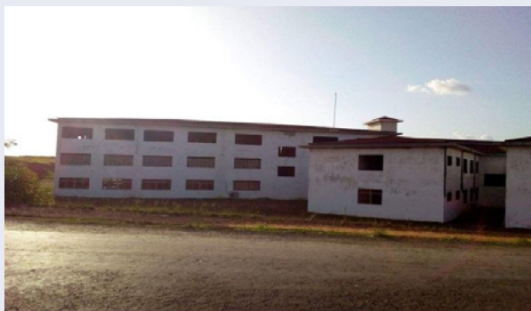
Bong Community College under construction
