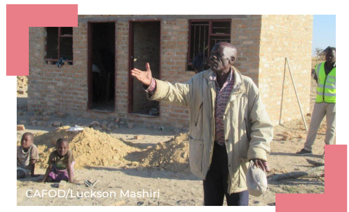
Caritas Harare shelter project following Cyclone Idai Zimbabwe
