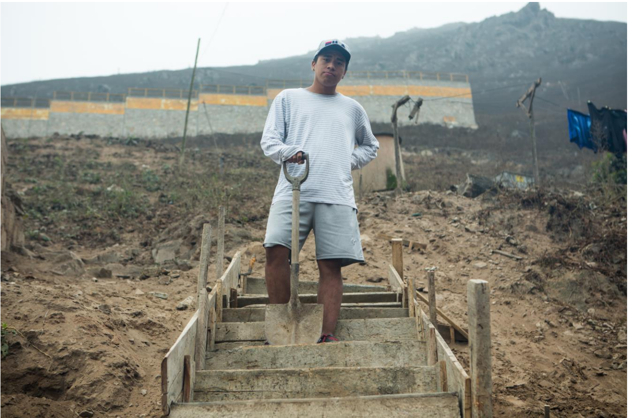
Paolo, building a staircase, with a retention wall in the background.
