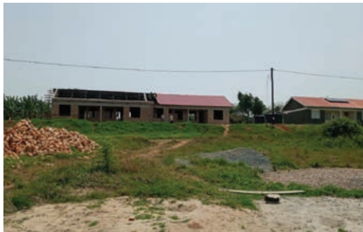
Construction of school in Uganda
