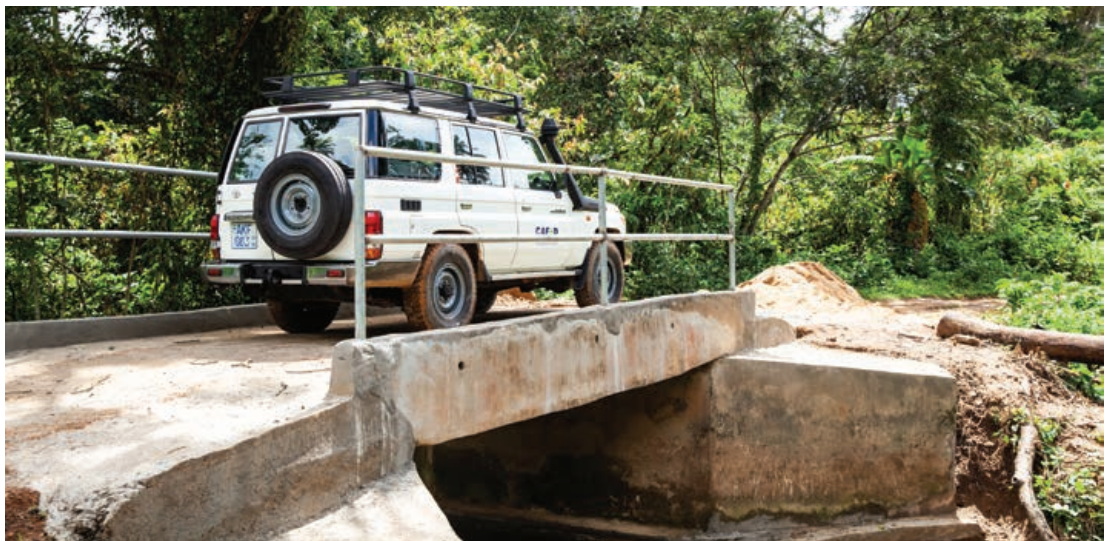
The rebuilt bridge, Sierra Leone
