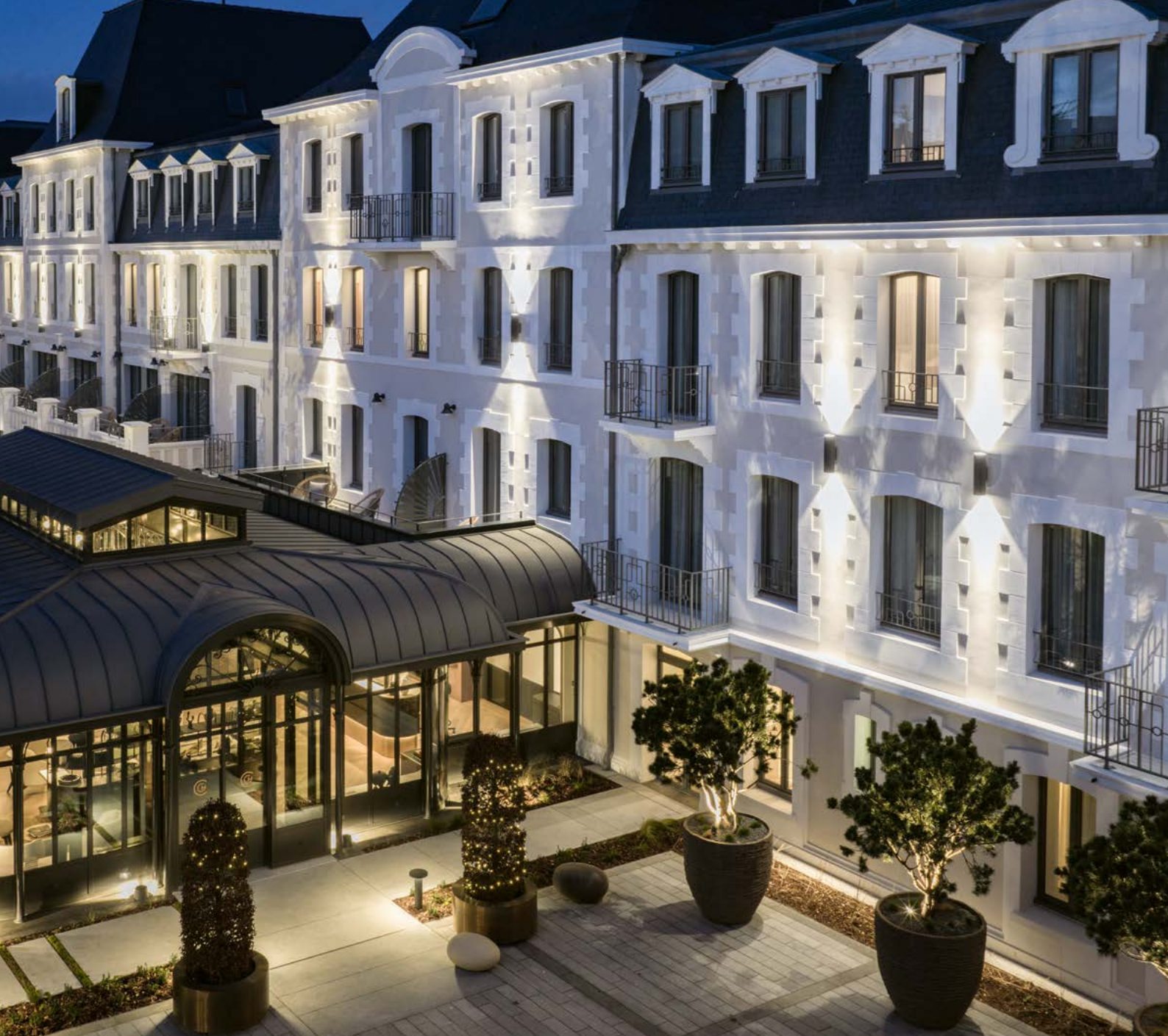
Closely coordinated lighting of the building and its surroundings underscores the high quality of the Grand Hôtel de Courtoisville – Saint-Malo, France.
