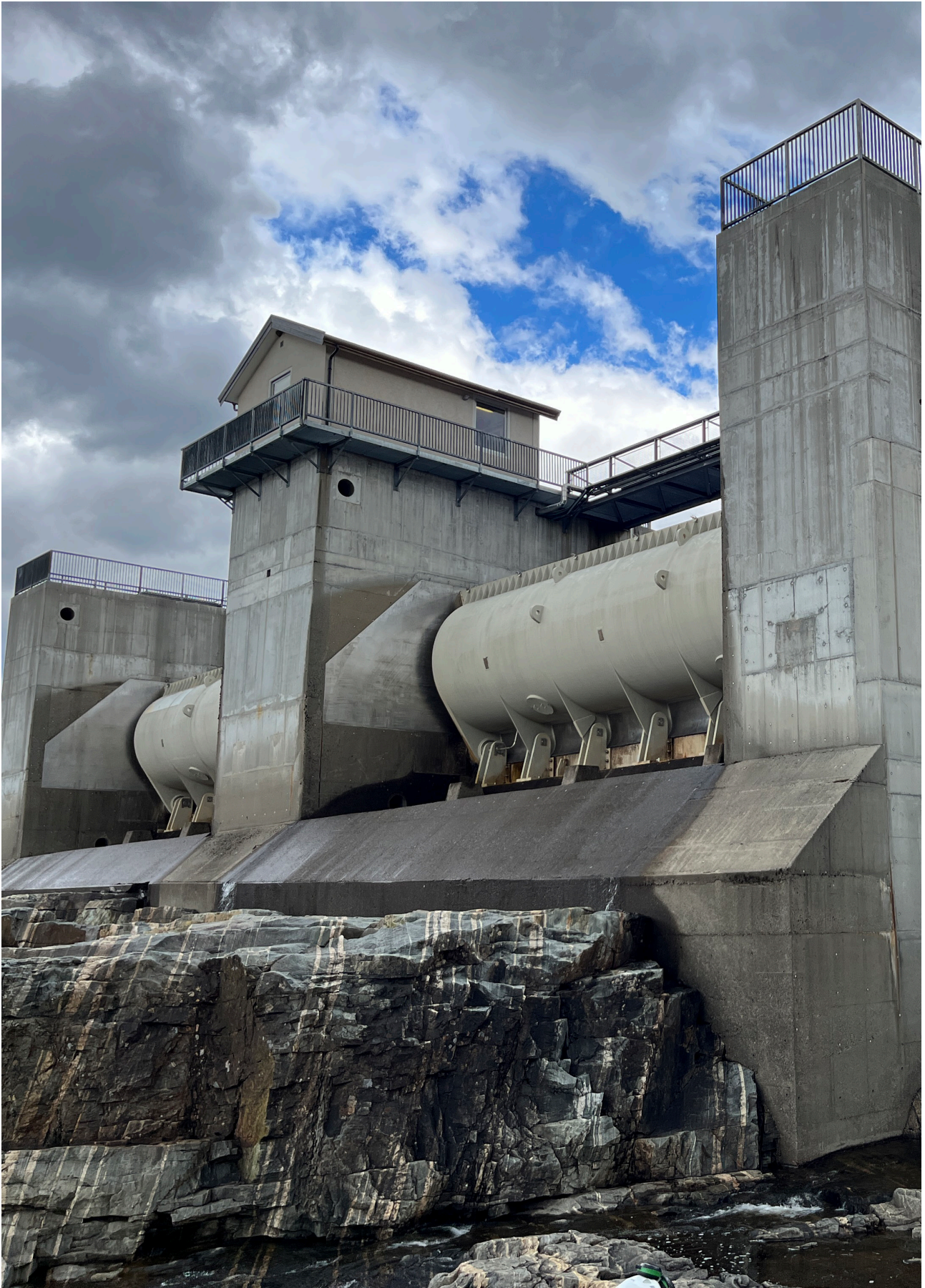
Site inspection at Aunfoss power plant in the Namsen River
