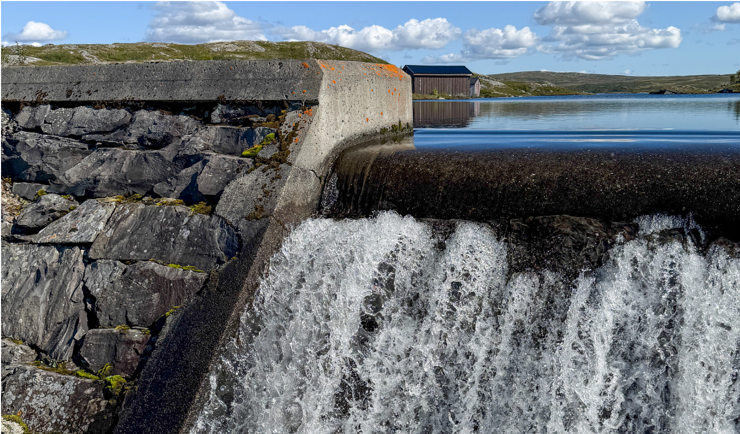
Dam facility at Skurdalssjøen
