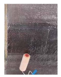
In situations where conventional strengthening systems such as external post tensioning, section enlargement or general repairs will not provide the necessary support, Carbon Fiber Reinforced Polymer (CFRP) systems can often be the solution. The above pictures show an industrial structure getting a flexural upgrade with the use of CFRP fabric.
