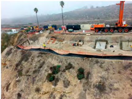
SLOPE STABILIZATION USING DYWIDAG STRAND ANCHOR SYSTEM AND DYWIDAG DYNA FORCE® SYSTEM - PASEO DEL MAR ROAD AT THE WHITE POINT NATURE PRESERVE IN SAN PEDRO, CA.
